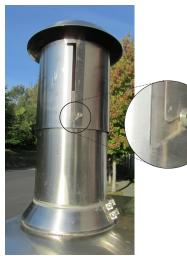
Flue extended and locked.
