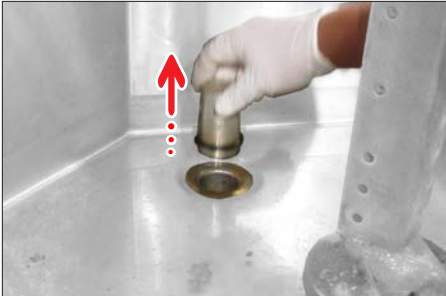
Lift out Drain Stand Pipe.
